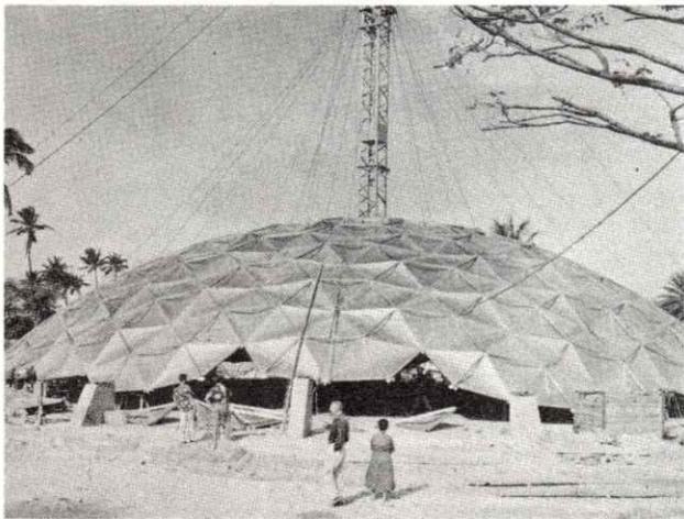
Fig. No. 99 Central mast erection technique Kaiser dome Figs. 79, 80, 81. Compressive and tensile characteristics of aluminum permit a semi-stress reversal in components during erection. Advantages similar to pneumatic technique of Fig. 97. Plywood dome Figs 43, 44, 45 and 46 erection similar.
