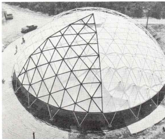
Fig. No. 21 One hundred twenty foot diameter strut and membrane dome. An 8^V Triacon breakdown, vertex zenith truncated along pent-cap. Struts have square flange ends bolt to cylinder ring, pull chain to membrane secures and adjusts membrane tension. A Synergetics Incorporated project.
