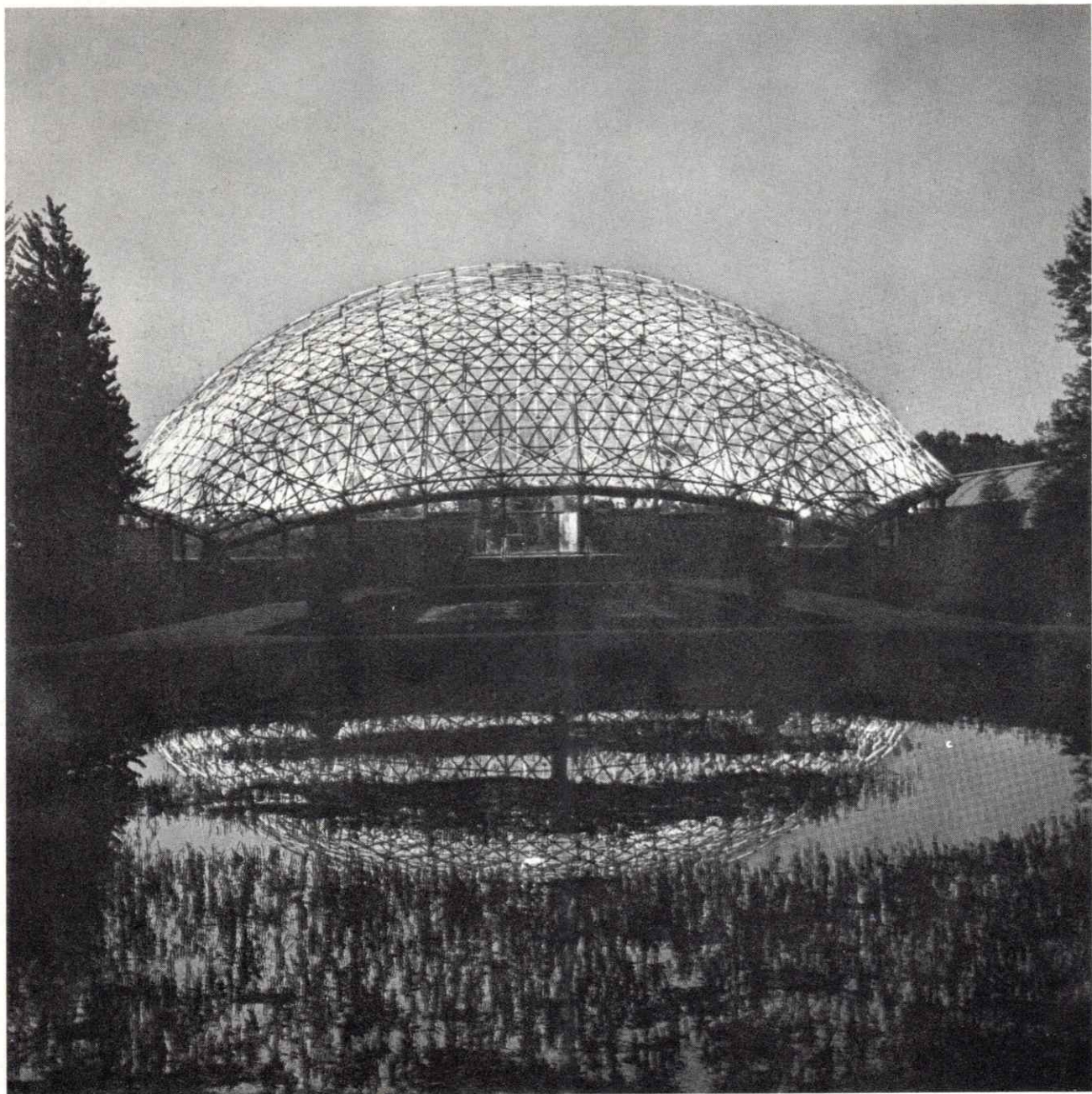
Fig. No. 73 Climatron at the Missouri Botanical Gardens in St. Louis, 175' diameter dome. Similar breakdown and frequency as ASM dome.
