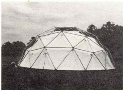
Fig. No. 103 Assembly sequence 55' diameter strut and membrane 3 V Alternate dome. Note suspension sequence and pull chain adjustment at vertex casting.
