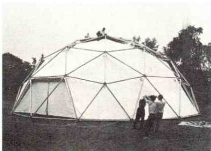
Fig. No. 103 Assembly sequence 55' diameter strut and membrane 3 V Alternate dome. Note suspension sequence and pull chain adjustment at vertex casting.
