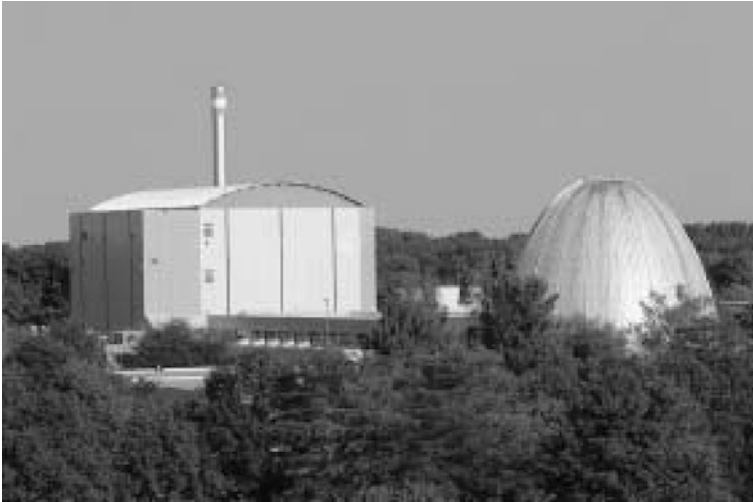
Fig. 1.6 Egg-shaped research reactor (“Atomei”) in Garching near Munich. In the building on the left the new research reactor FRM II, completed in 2004, is located ( photo Albert Scharger/TU Munich)
