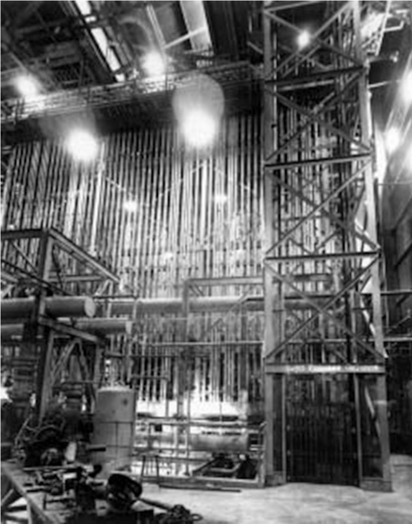
Fig. 5.7 Thermal diffusion: a small part of the thermal-diffusion plant constructed during the Manhattan Project in Oak Ridge in the American Federal State of Tennessee. We can see the separation columns for the enrichment of the uranium isotope ^{235}\text{U} based on the principle invented by Klaus Clusius ( photo AEC photo of Ed Westcott)
