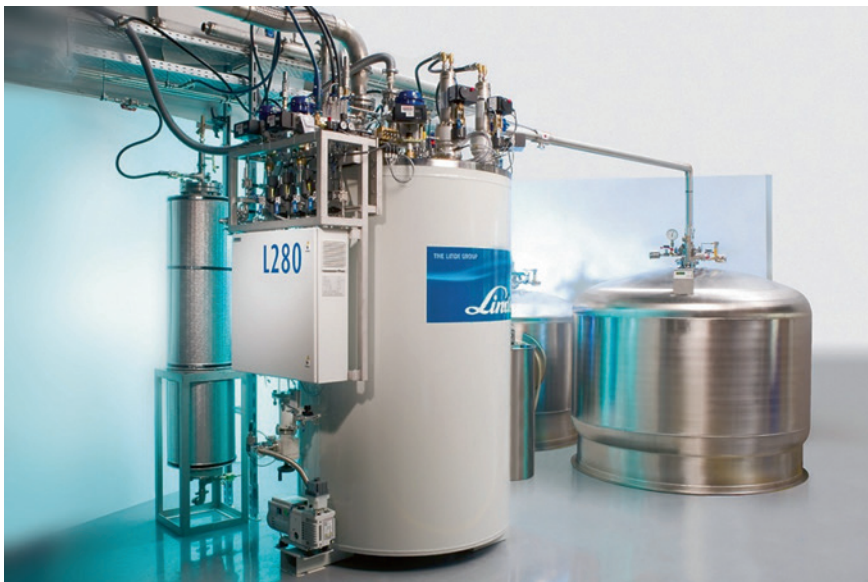
Fig. 1.3 Modern plant for liquefying the noble gas helium. On the left we see the controls and the cold box of the liquefier, on the right the storage vessel for liquid helium ( photo Linde AG )
